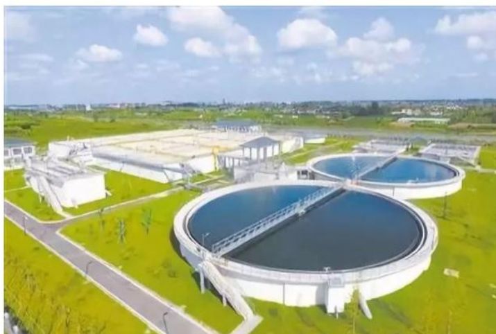
工厂污水全经污水处理 All factory's water through sewage treatment
