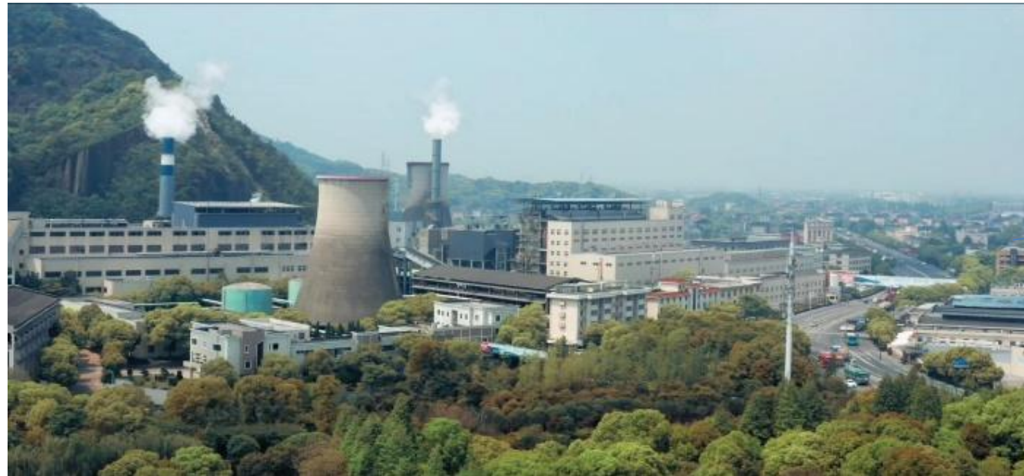
'City steam' – Combined Heat and Power Thermal Plant
